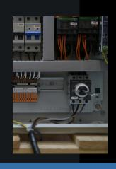
SIZE: The enclosure is mild steel by Schneider, 500mm high, 400mm wide and 200mm deep for a dual pump DOL, with a door interlocked isolator.
