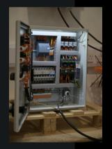
IMPROVED CONTROL: Overload reset buttons included as standard. Enhanced pump management (e.g. when pump one is turned 'off' then pump two stays as the duty pump)
